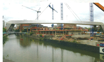
The footbridge being craned into position.
