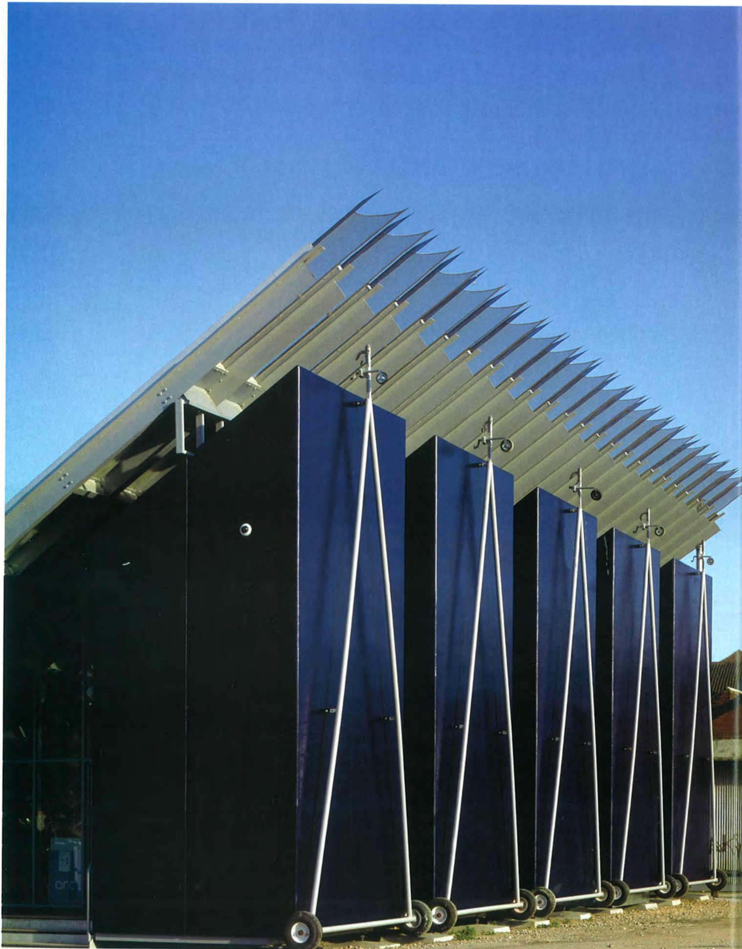
Hull is home to a big caravan manufacturer, a fact alluded to by the wheels and tow bars and the bulbous plastic windows in the sides of the pods.
