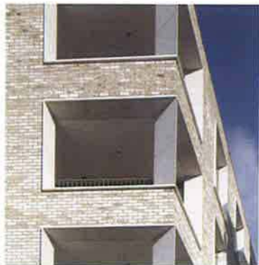
3. Precast GRC fins stand at the corner of each balcony
