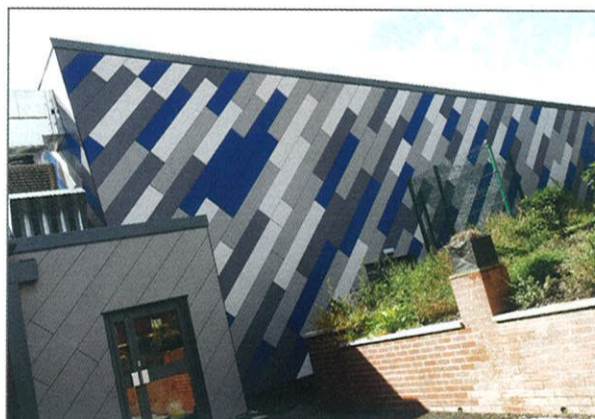
The Marley Eternit rainscreen cladding insulation solution specified on Prestwich Arts College achieves an overall wall U value of 0.19 W/m2K.
