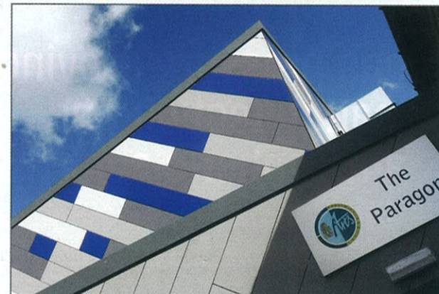
The durable and lightweight nature of Marley Eternit's fibre cement rainscreen cladding allows the creation of more visually engaging structures.
