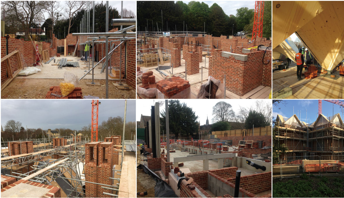
建築結構施作過程 THE PROCESS OF BUILDING CONSTRUCTION
