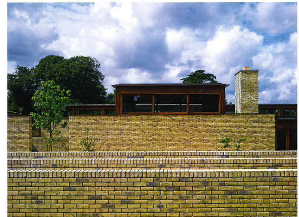
The building is made from a collection of timber lanterns set within old garden walls, creating a sequence of courts, orchards and lawns all linked together.
