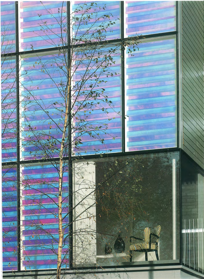
colours of the facade change as quickly as the light, making the flats the focus of the street.
