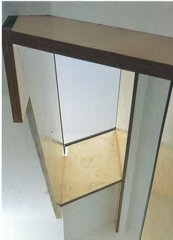
Solid ply is used to box in the staircases.
