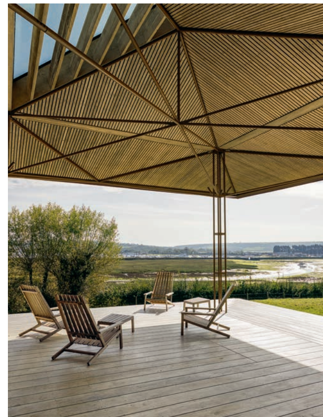
VERANDA The delicate steel superstructure and the timber-lined roof almost appear to float above the accoya-wood decking, which is furnished with 'Between Lines' chairs designed by Stine Weigelt
